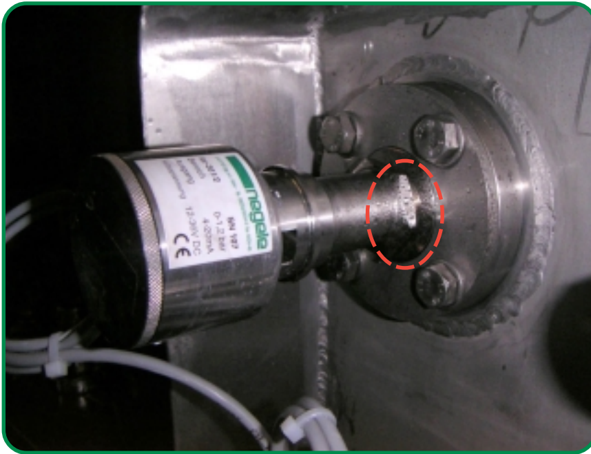
Pic. 1: Condensation at the level sensor LAR-361
