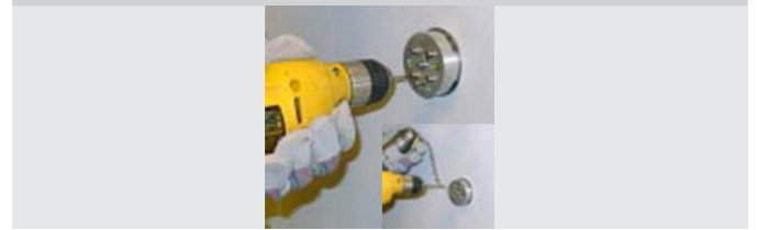
Figure 5-21 Drill more mounting holes
