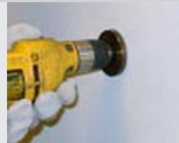
Figure 5-17 Prepare surface with grinder
