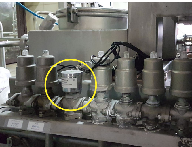
NCS-11 installed at one of the Brewery Plant in south
