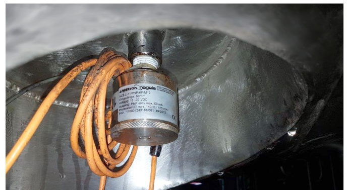
NCS on the bottom of Flash Pasteurizer Tank
