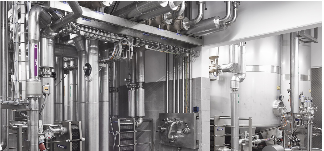
The CIP system with active phase separation by means of sensor technology
