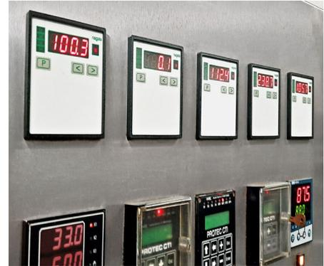
The digital local display DPM could be installed in the existing openings of the predecessor equipment.
