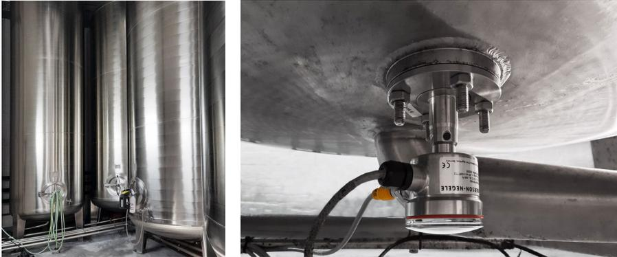
The high measuring accuracy of  $\pm 0.15\%$ , a response time of  $< 0.2$  seconds and the integrated density compensation make the D3 ideal for high-precision level control in brewery pressure tanks, even with temperature changes or rapid volume changes such as during filling.
