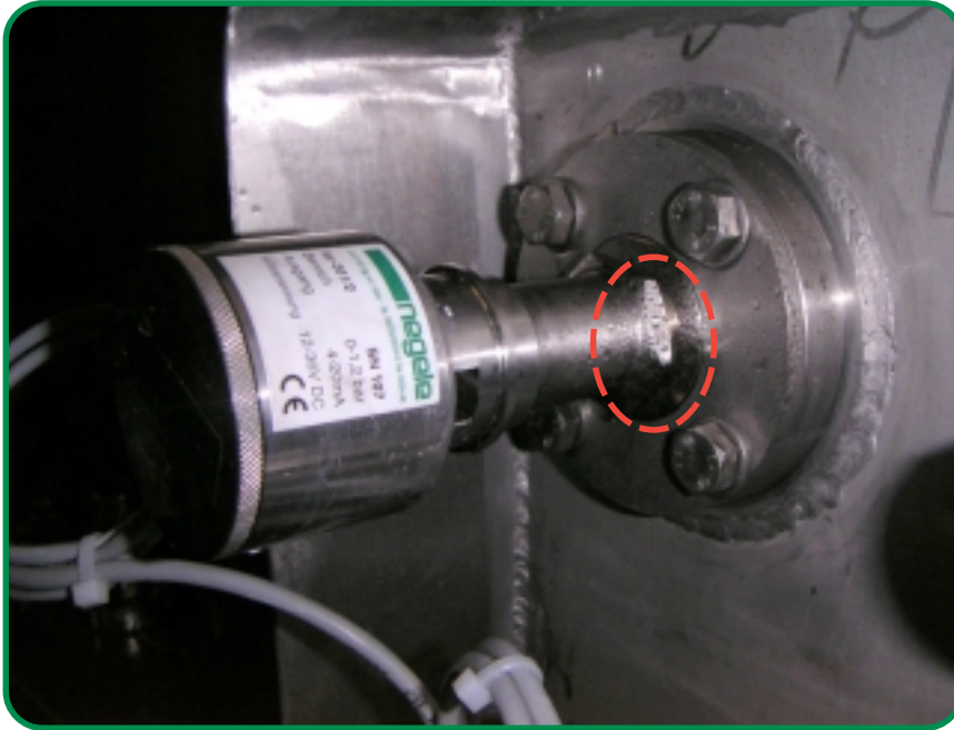
Pic. 1: Condensation at the level sensor LAR-361
